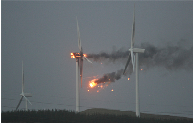
Fig. 5. Wind turbine fire at Ardrossan wind farm [17].
